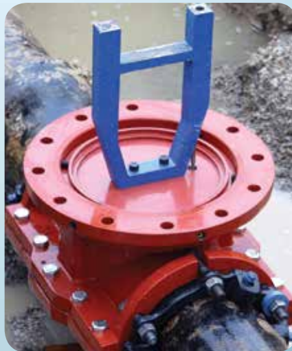
Internal equalization completion plug installed.
