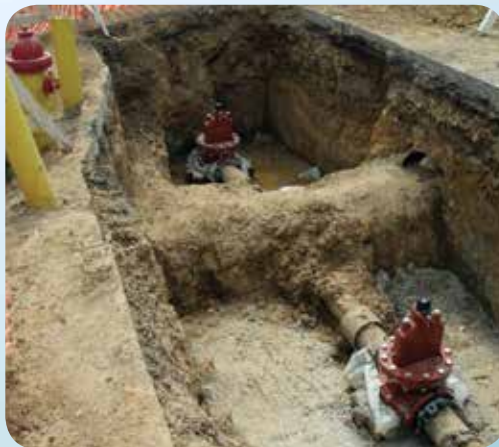
InsertValves on AC pipe for main control and hydrant replacement preventing asbestos fibers becoming airborne.
